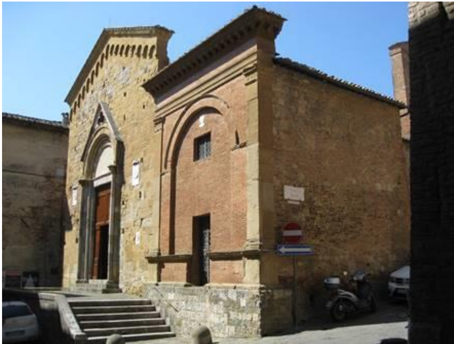
San Pietro alla Magione with its later brickbuilt extension on the right
