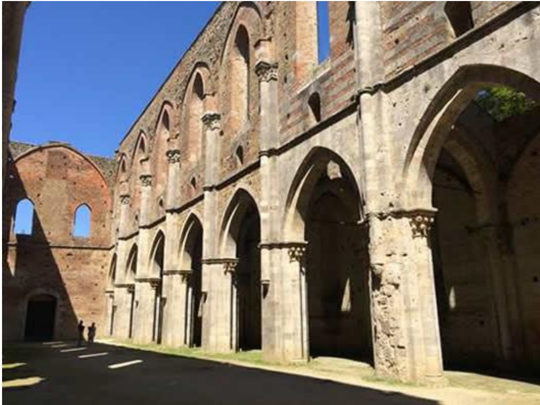
The roofless remains of the great abbey church
