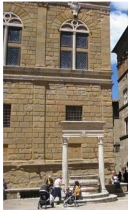
The well with the Palazzo Piccolomini behind
