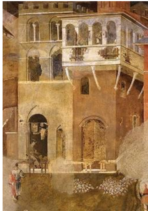
Bad Government with broken buildings
